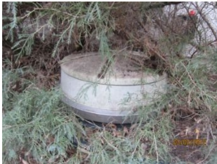
Noted: Lift station for sewer line to pump sewage up to the main sewer line. This is not a part of the home inspection.
